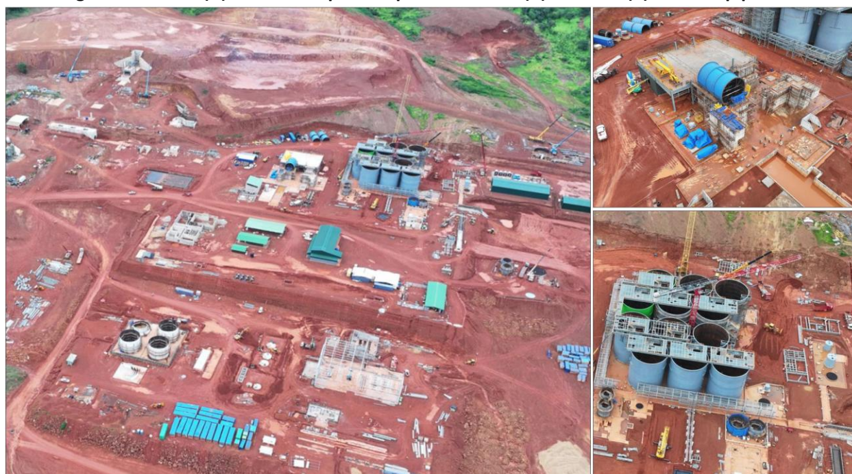
Figure 1: Kiniero (A) aerial view process plant and infra (B) SAG mill (C) CIL with pipe rack
