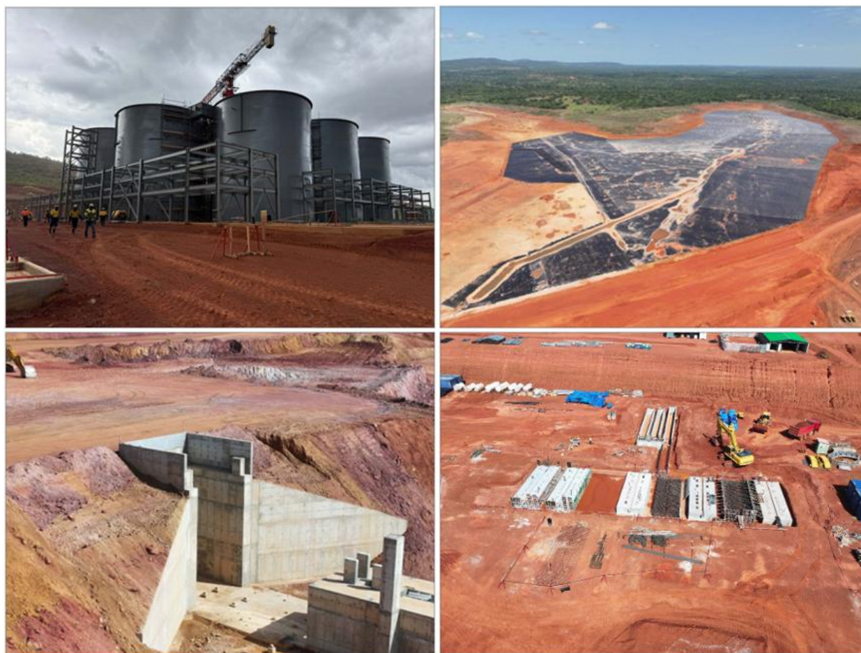
Figure 2: (A) CIL with main pipe rack (B) tailings storage facility (C) primary crusher ROM pad and chamber (D) power station generator bases
